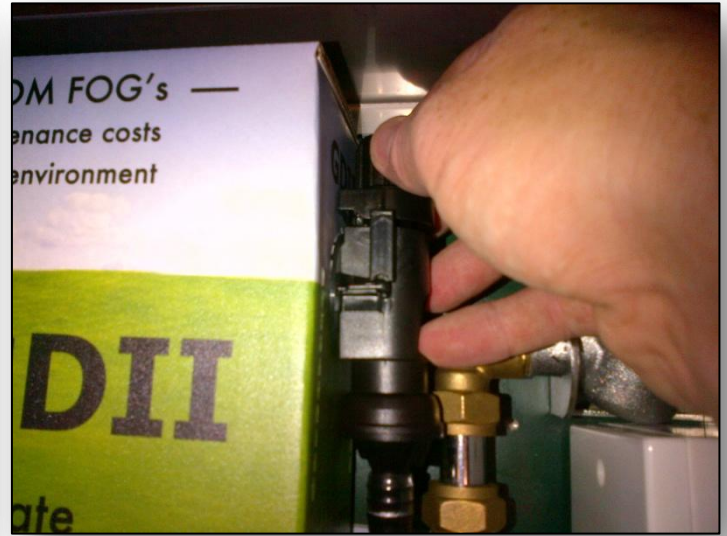
Step 6: Attach the connector from the GDII over the bag in box tap
