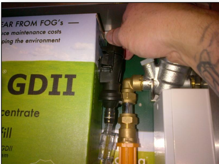
Step 7: Tighten connector
